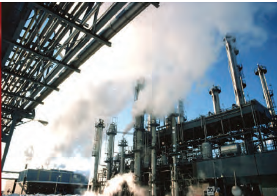
Instrumentation and Automated Pneumatic Controls
